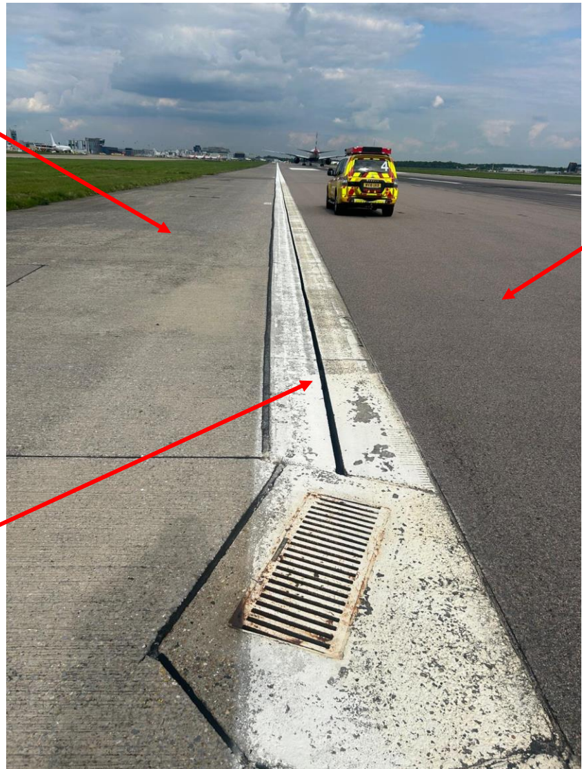
Photo 1: Existing Northern Runway showing the existing slot drain
